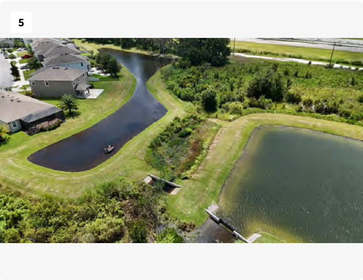
Pond P1 - At normal holding capacity, all water control structures are clear.
