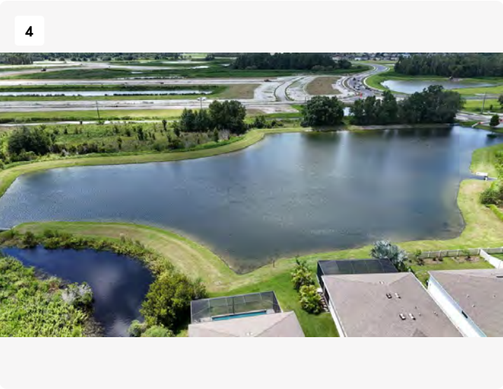
Pond O - At normal holding capacity. Techs treated for Torpedo grass and minor Pennywort along the shore.
